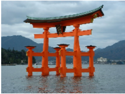
Fig.1 Grand Gate of Itsukushima Shrine: Typical column-Nuki joint
