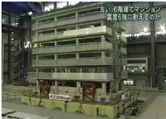
Shaking Table Test for full scale six-story RC building (TV Asahi)
